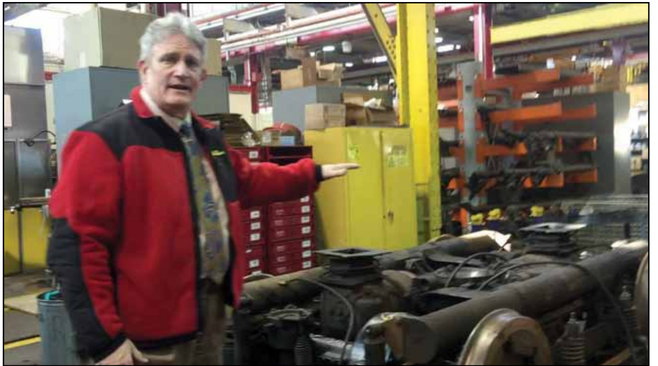
Edward Belanger, maintenance supervisor of the MBTA’s subway main repair facility in Everett, explains the components of the “truck” that is the propulsion unit that sits under the Mattapan PCC cars. On average, the MBTA repair crews receive one truck per month to re-build or repair. Bill Forry photo
