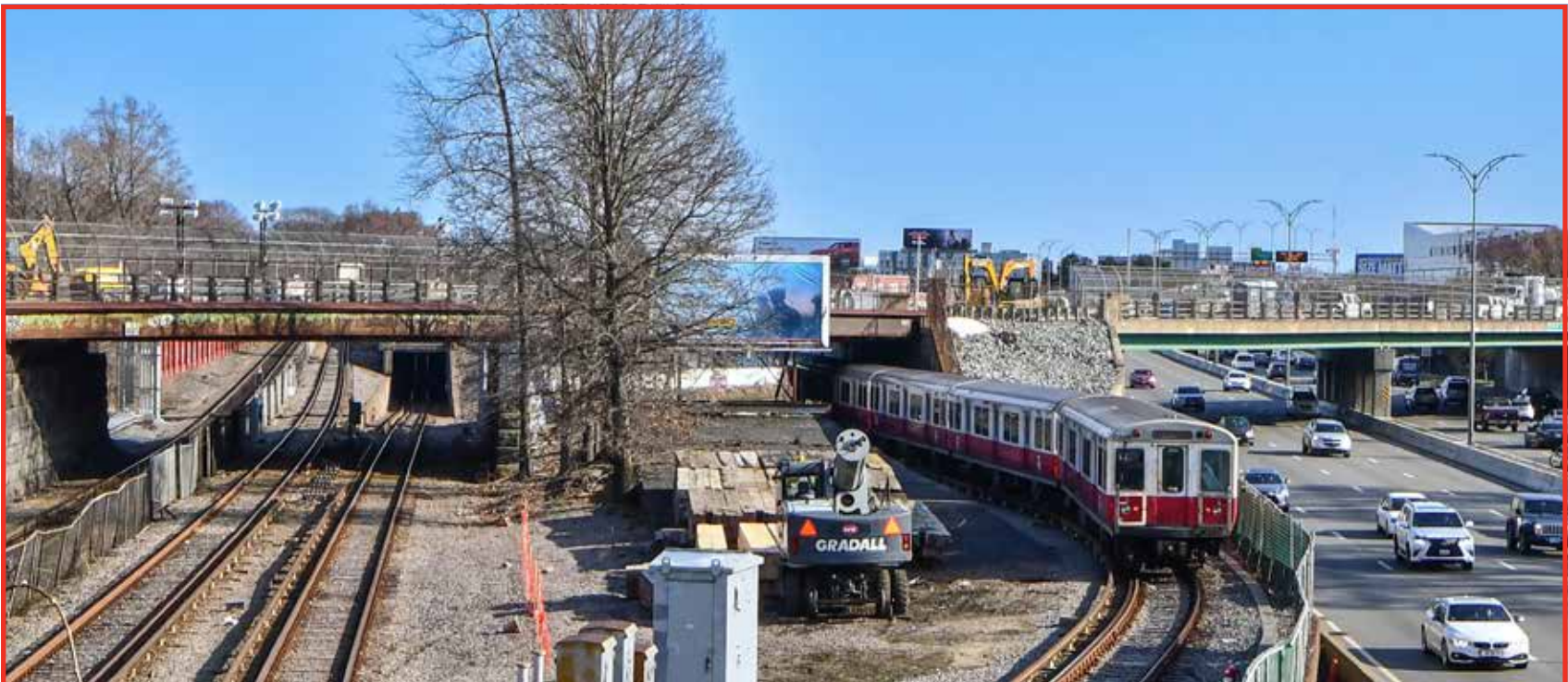
Red Line passing under Dorchester Avenue Bridge while under construction
