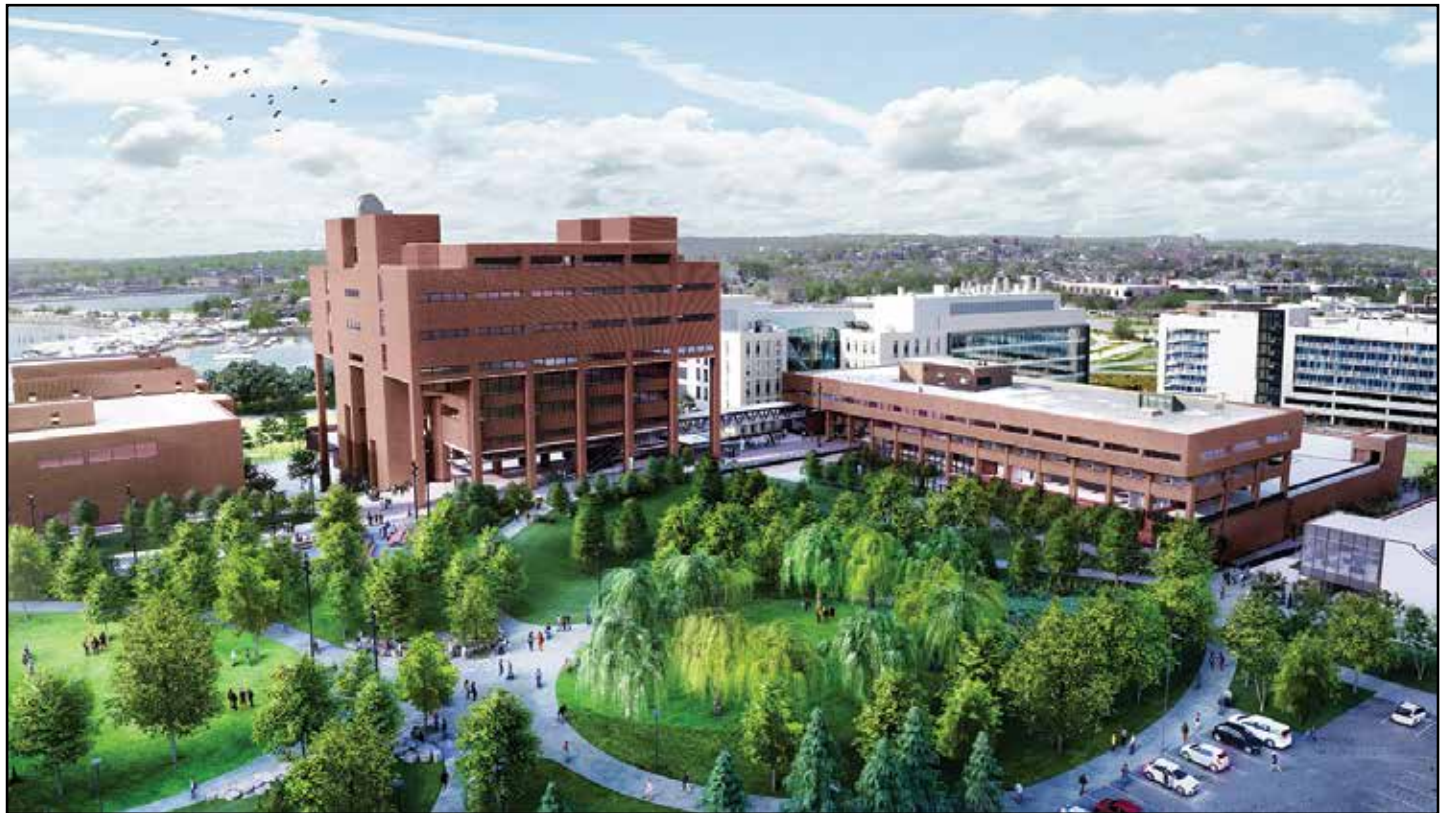
The rendering above shows what the fully completed Quad on the UMass Boston campus will look like with mature trees and vegetation. The green space and walking paths have replaced what was a former Science center building and a desolate, concrete plaza that covered a parking garage that had long been closed off because of structural defects that made it unsafe. At right, UMass Boston Chancellor Marcelo Suárez-Orozco greeted visitors in the simulation lab at the Manning College of Nursing and Health Sciences during the announcement of $3 million in funding sponsored by Rep. Lynch earlier this year.
