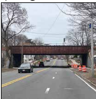
The MBTA bridge over Gallivan Boulevard. Reporter file photo
