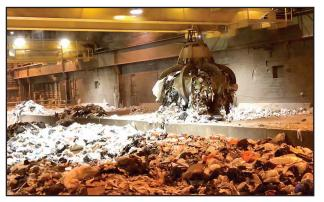
A grapple crane inside a processing facility in Haverhill, Mass. prepares to move waste to the incinerator. Photo courtesy Covanta
