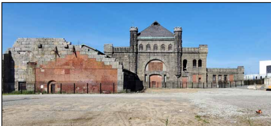
The iconic Calf Pasture Pumping Station on Columbia Point. Boston Landmarks Commission photo The iconic Calf Pasture Pumping Station on Columbia Point. Boston Landmarks Commission photo
