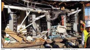
The damaged signal bungalow at JFK-UMass station is shown in this photo taken on the day after the June 11 derailment. *Image courtesy MassDOT*
