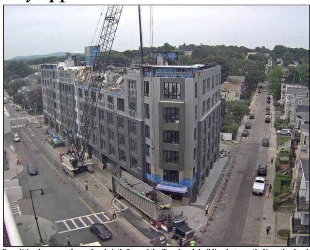
Demolition began on the roof and sixth floor of the Treadmark building last month. Now, the developer- Trinity Financial, Inc.- has won city approval for a plan to deconstruct the top five floors of the structure to make way for a rebuilding process that should take most of the next year to complete. Image courtesy Trinity Financial, Inc.
