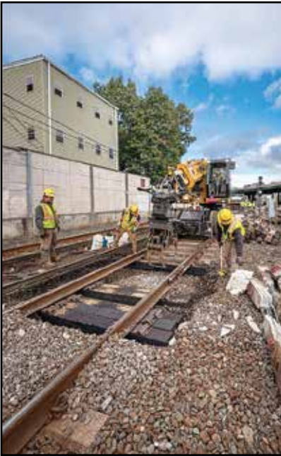
Workers replacing track along the right-of-way between JFK-UMass and Savin Hill stations last week. MBTA photo
