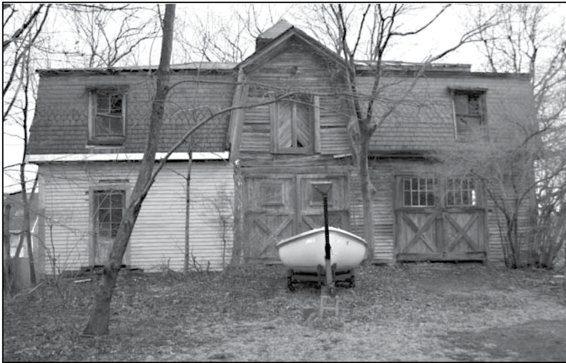
This two-story stable on the property at 24 Grampian Way was built in 1873 and was later used to house a squash court used by sporting goods pioneer George Wright, according to a new report for the Boston Landmarks Commission.
