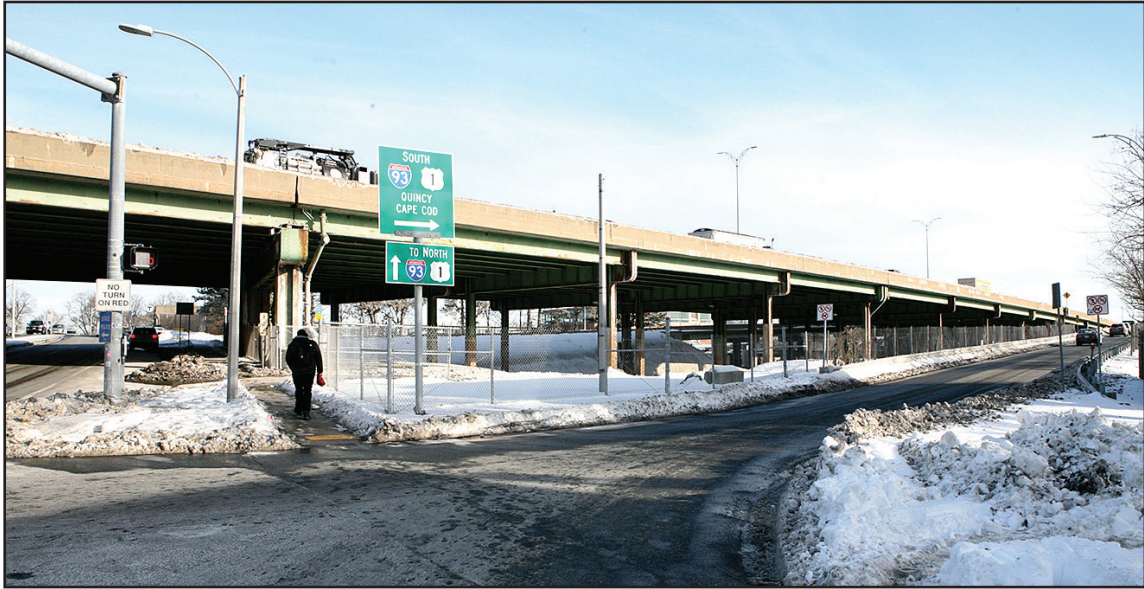
A state highway project long in the works for I-93 abutting Columbia/ Savin Hill surprised many by moving quickly to the construction phase this spring. Seth Daniel photo
