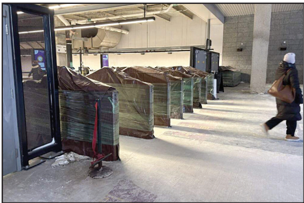
The idle fare gates at the tracks at South Station. are under cover, they are exposed to the bitter cold that has affected some of the T’s train and subway operations over the last week. On Monday morning, the gates were left wide open to let passengers through without scanning a ticket. Users on Reddit were posting Saturday about the gates similarly being out of use and covered. The T began on Dec. 30 to require commuter rail passengers to tap or scan a train ticket to enter the track area at South Station and to require
