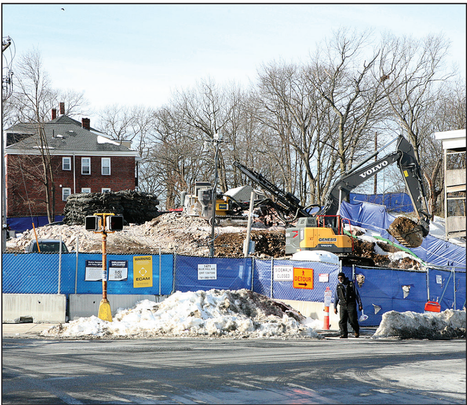
The site at 1471 Blue Hill Ave. as seen on Monday this week. A California-based development firm is building a structure that will include 44 units of rental housing. Seth Daniel photo
